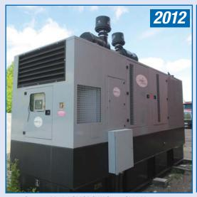
2012 Somers Model SMGDCWAS800 Skid Mount 1,000 KVA, 347/600V Generator, s/n SC620803-84UG p/w Cummins Model QSG23-G3, 1,200 HP Diesel Engine, s/n 00316079 (less than 100 hours)
